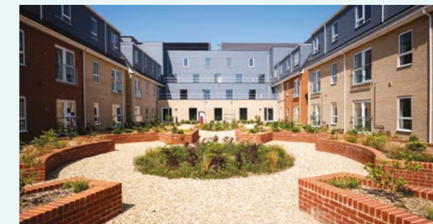
Ashey Road – Ryde, Isle of Wight £12.0m Gross Dev Value (net of Grant) Extra care and shared ownership for over 55s, or over 45s with a support need 27 x 2-bed bungalows, 75 x 1- & 2-bed apartments c.150 people housed
