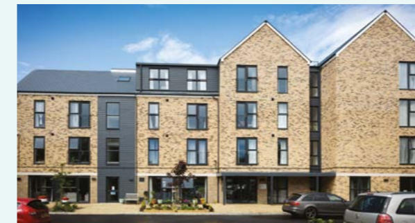
Colwell Road – Freshwater, Isle of Wight £10.3m Gross Dev Value (net of Grant) Extra care and shared ownership for over 55s, or over 45s with a support need 75 x 1- & 2-bed apartments c.110 people housed
